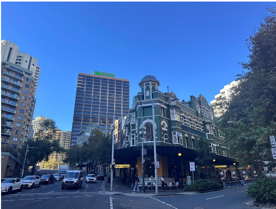
Figure 5: 40-44 Wentworth Avenue, and Wentworth Avenue streetscape, looking north
