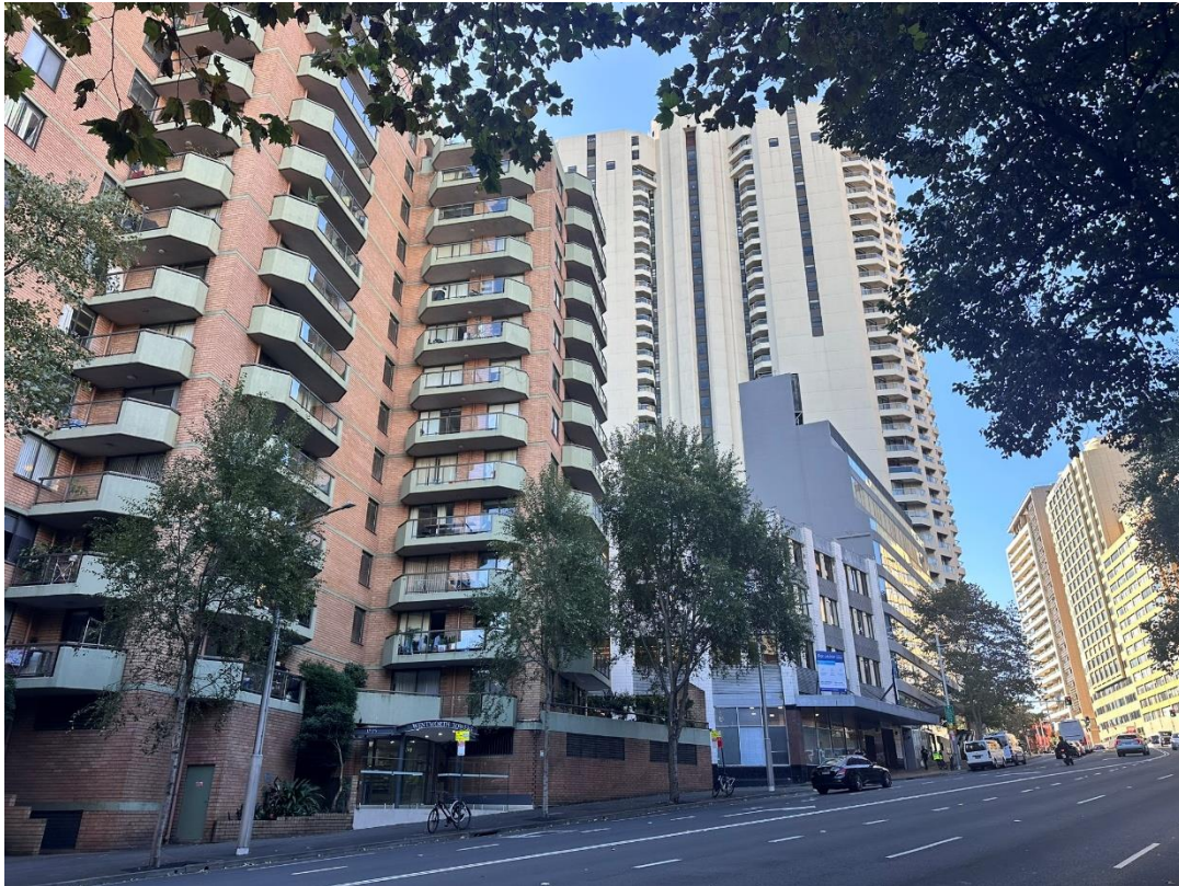
Figure 6: Wentworth Avenue development directly opposite the site, looking north-west
