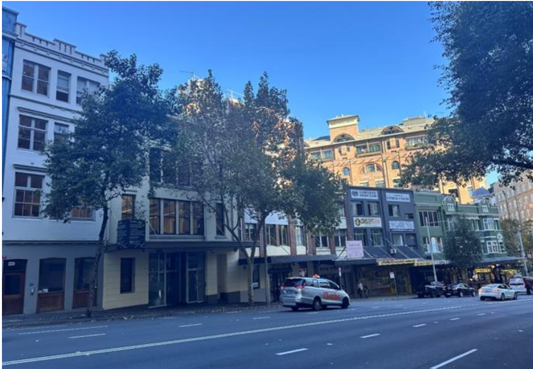
Figure 4: Heritage listed warehouses 24-44 Wentworth Avenue (directly south of the subject site), looking south-east
